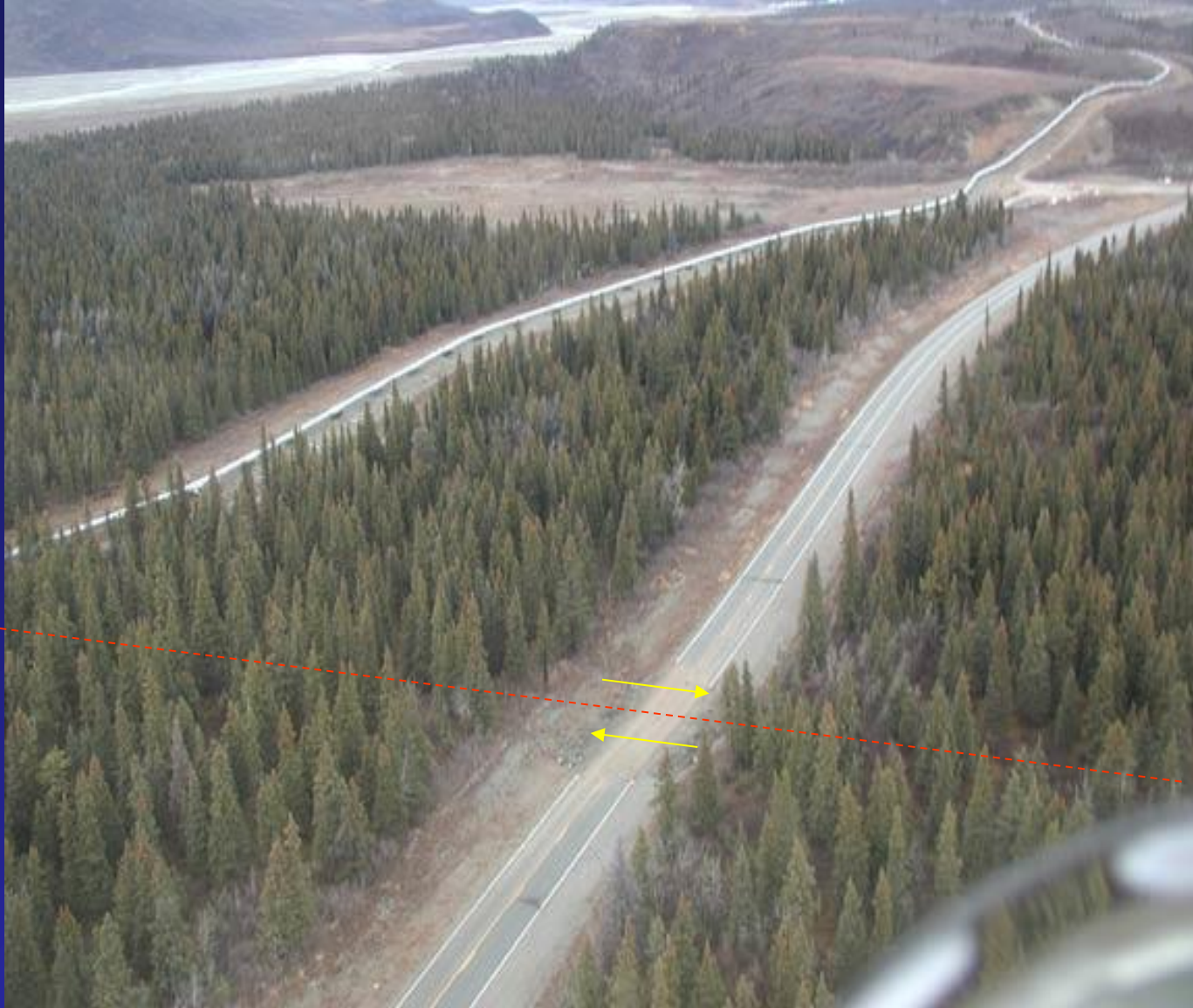
M 7.9 Denali fault, Alaska, earthquake of November 3, 2002. Milepost 215.5 on the Richardson Highway ( http://earthquake.usgs.gov/eqinthenews/2002/uslbbbl/photos/pr071102/rhnpipeline2.jpg )
