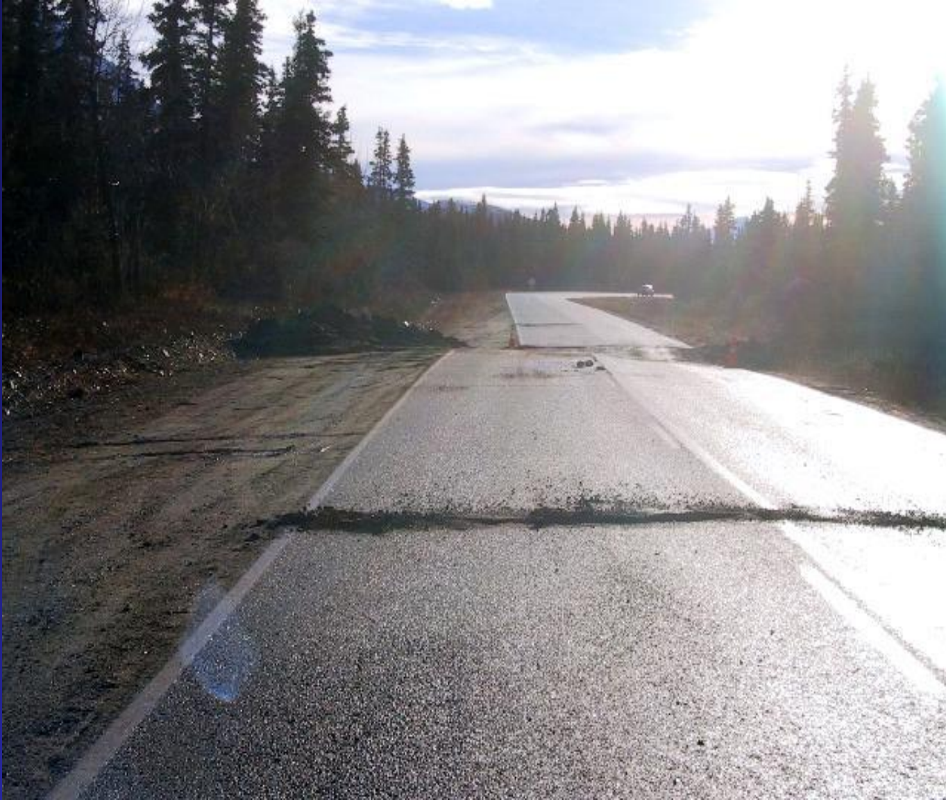
M 7.9 Denali fault, Alaska, earthquake of November 3, 2002. Milepost 215.5 on the Richardson Highway. The direction of view is approximately from north to south. The fault trace is running almost NW-SE direction. The horizontal offset is approximately 2-2.5m. Photo courtesy: Akihiko Ito
